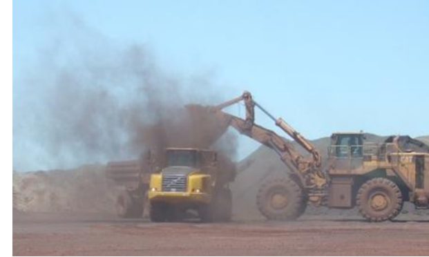
Material handling dust FDR 2 impacting outside of work area
