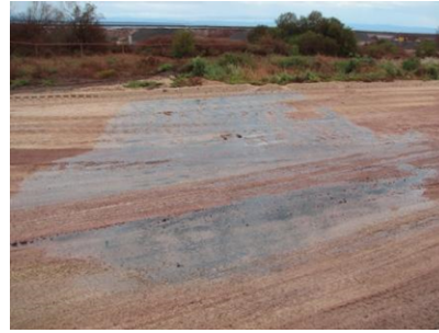
Hydraulic oil leak from truck
