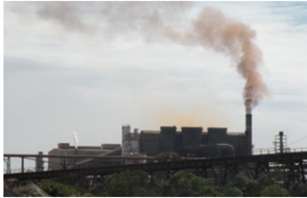
Pollution control equipment not functioning
